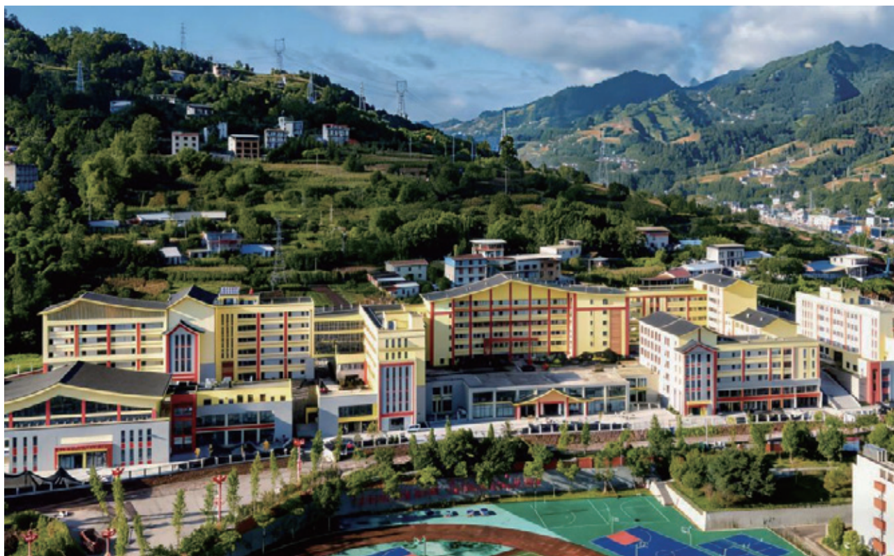
Pension finance: Sichuan Branch supported the Regional Elderly Care Center Project in Xiaoliangshan, Mabian Yi Autonomous County
